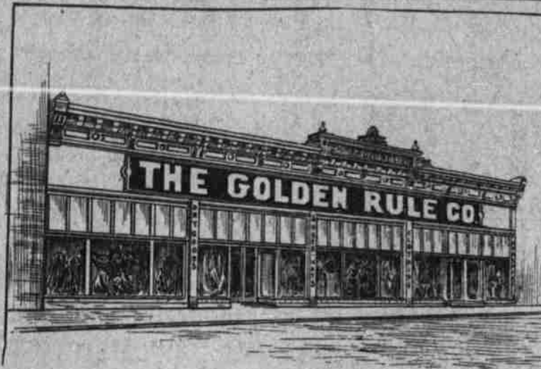
Golden Rule Company's Store which is not large enough to handle holiday goods. Room formerly occupied by S. H. Dalton has been leased for the annex.
