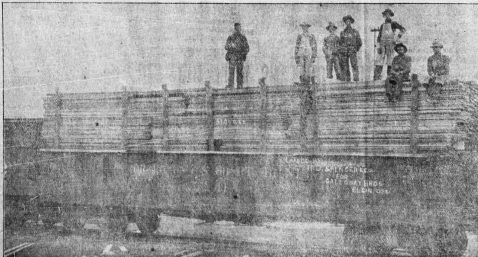
Next to the Largest Load of Lumber Ever Loaded in the World. This was Loaded At Elgin.
