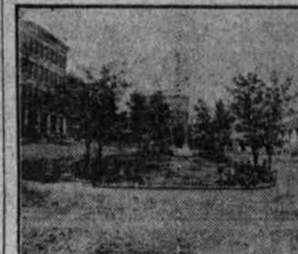
A NEAT PIECE OF PARKING.
