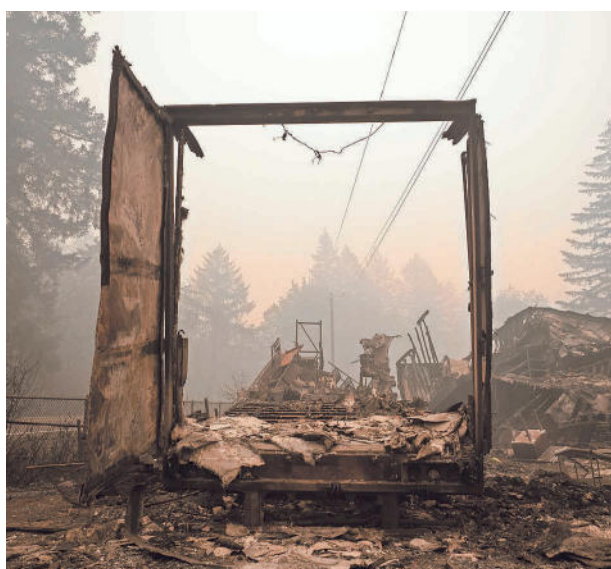
Images from Gates School and the former Beachie Creek Fire incident command post that was burned and forced to evacuate after new fires started on downed power lines. ANDY ADKINS / SPECIAL TO THE STATESMAN JOURNAL
