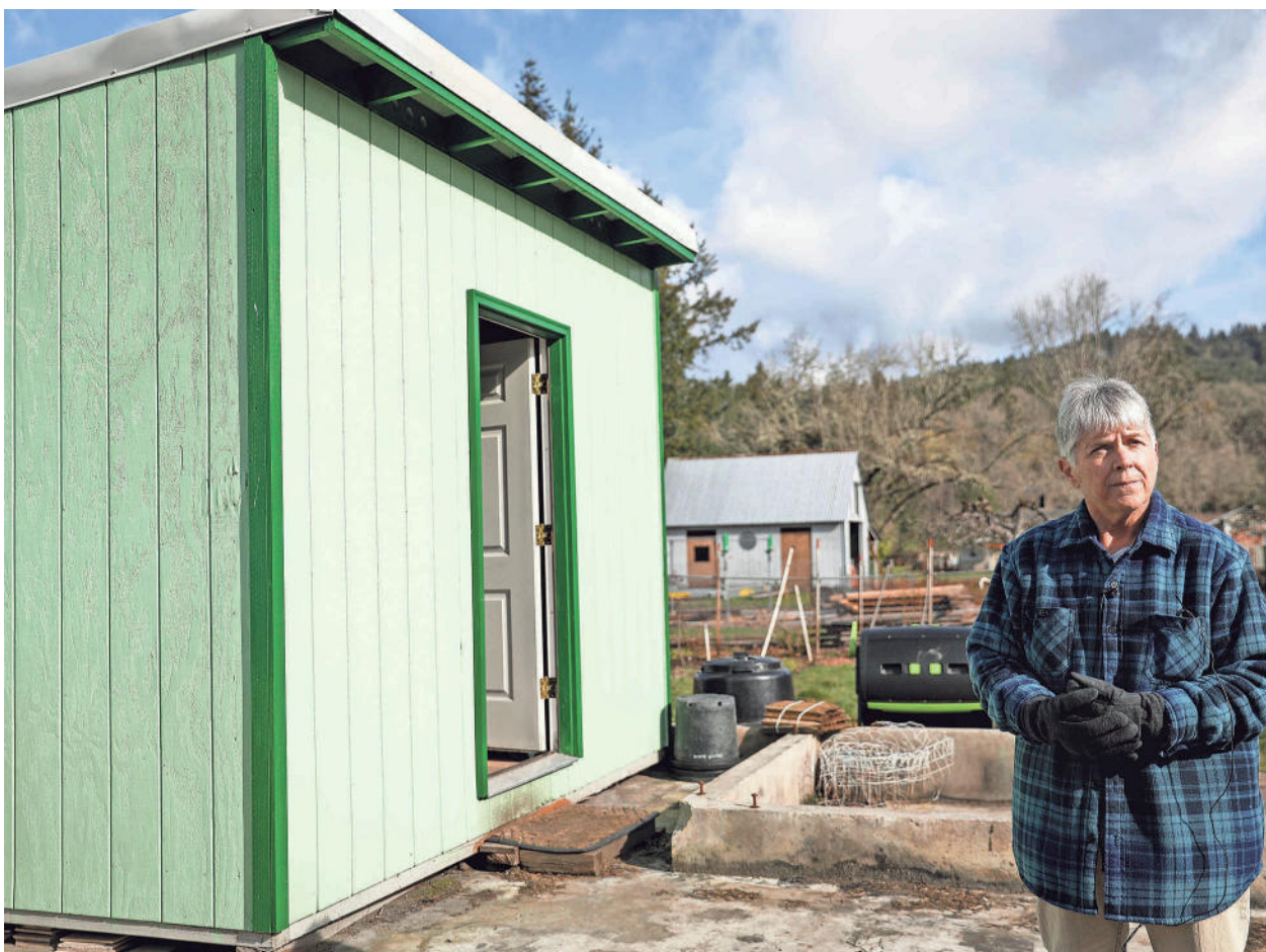
Above: Diana McGuire stores personal belongings in a shed she received through the project on Saturday in Lyons. McGuire's home and garage burned down in the Beachie Creek Fire. Top: Volunteer Tim Long builds sheds for Santiam Canyon residents who were affected by the fire on Saturday in Stayton. PHOTOS BY ABIGAIL DOLLINS/STATESMAN JOURNAL
