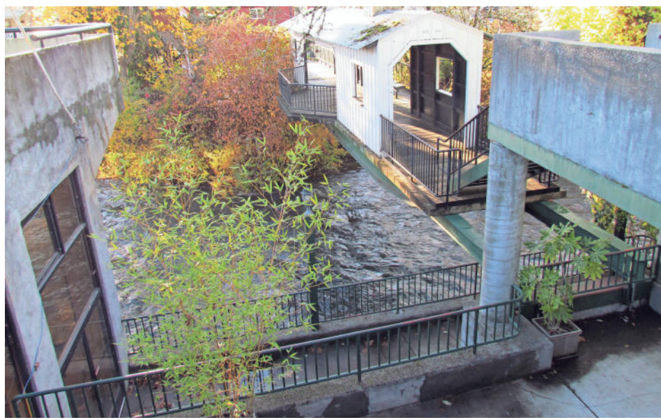
Water is a key element in Silverton's character, and a key focus of the city's infrastructure developments. JUSTIN MUCH | SILVERTON APPEAL TRIBUNE
