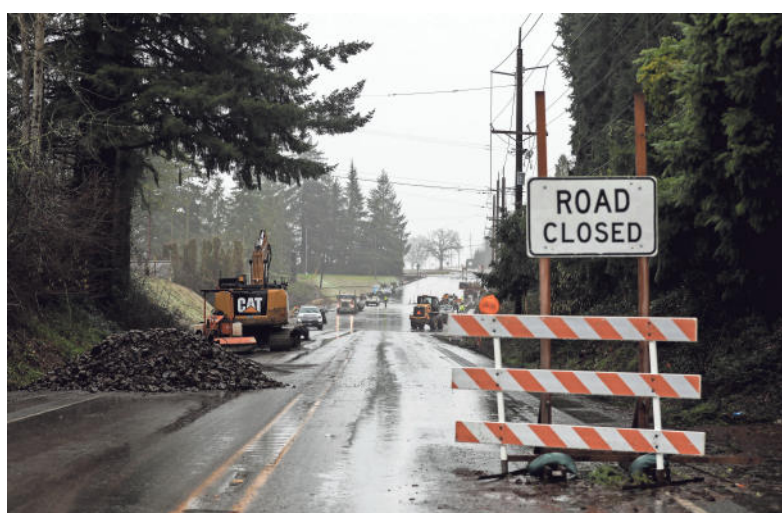
There are 395 bridges in Oregon in "poor" condition, according to 2020 data from the U.S. Department of Transportation.
