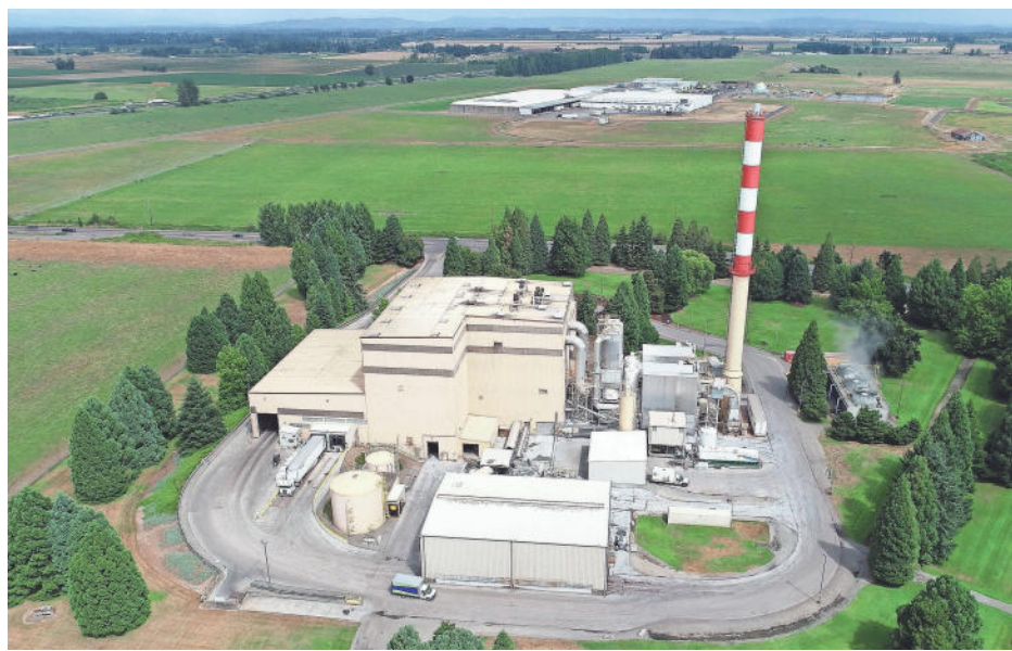
The Covanta Marion municipal waste incinerator facility in Brooks. DAVID DAVIS AND KELLY JORDAN/STATESMAN JOURNAL
