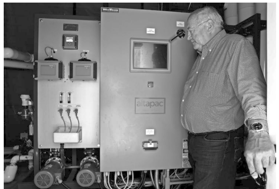
Detroit Mayor Jim Trett shows the temporary membrane water filtration system in Detroit, Oregon on Tuesday, May 11, 2021. BRIAN HAYES / STATESMAN JOURNAL
