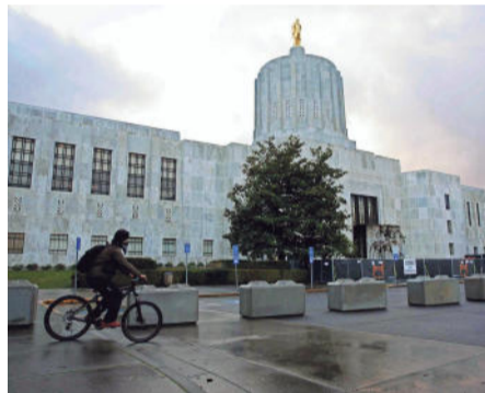
A man rides a bicycle past newly installed cement blocks placed outside the Oregon State Capitol Building in Salem on Wednesday, Dec. 30.
