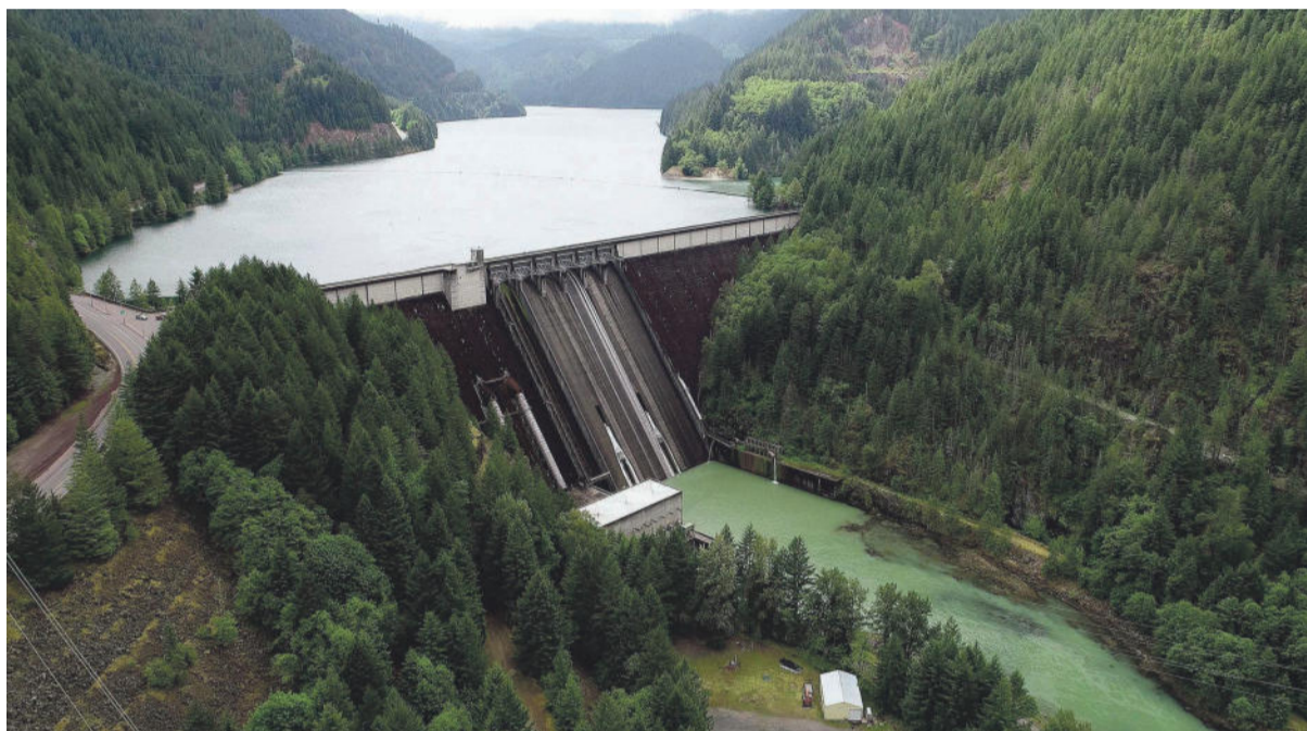
The Detroit Dam was constructed by the U.S. Army Corps of Engineers in the Willamette Valley and began operating in 1953. DAVID DAVIS AND KELLY JORDAN / STATESMAN JOURNAL
