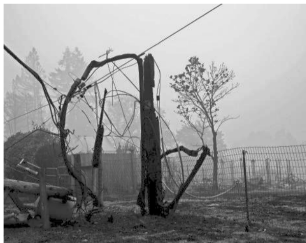
Damage to power lines from the Santiam Fire on Wednesday, Sept. 9 in Mill City, Ore.
