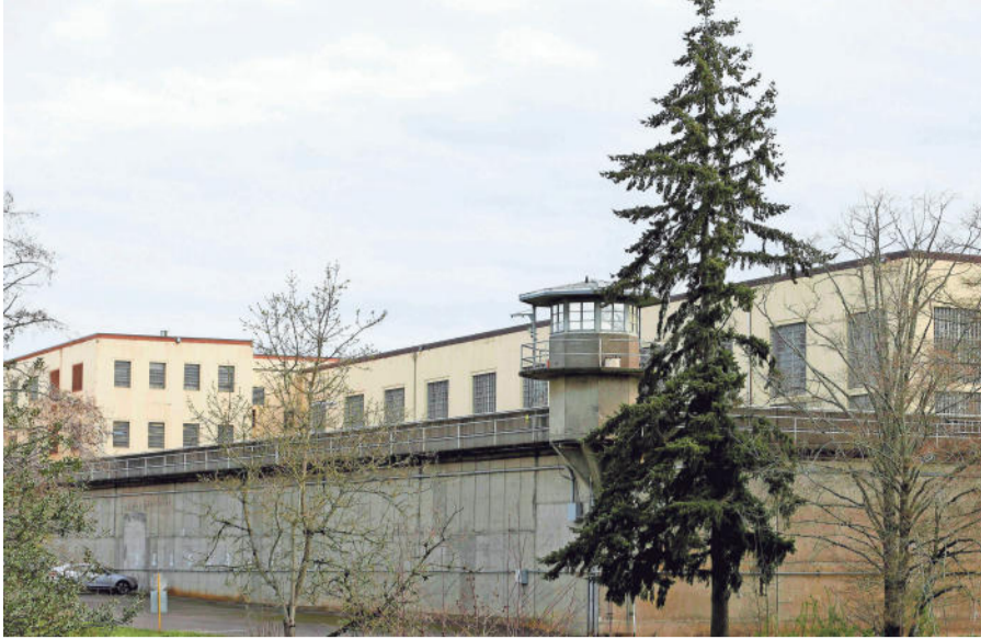
Tall concrete walls with guard towers surround the Oregon State Penitentiary, the state's only maximum-security prison, along State Street in Salem.
