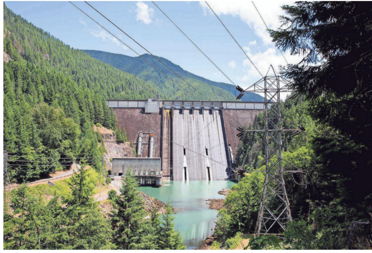
The Detroit Dam on the North Santiam River was constructed in 1953. STATESMAN JOURNAL FILE
