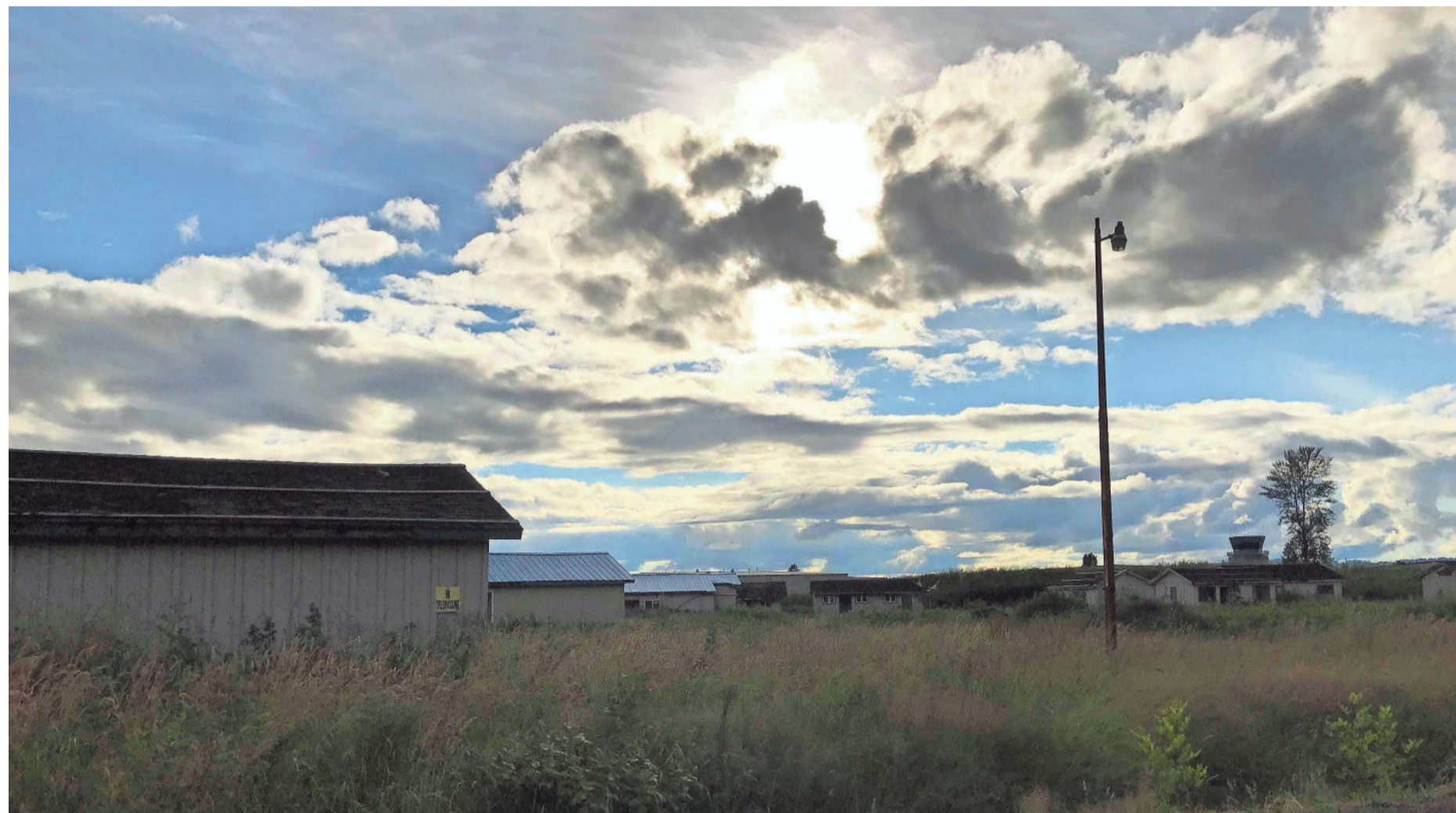
The former church camp bordering the Aurora State Airport has been abandoned for decades. BILL POEHLER | STATESMAN JOURNAL
