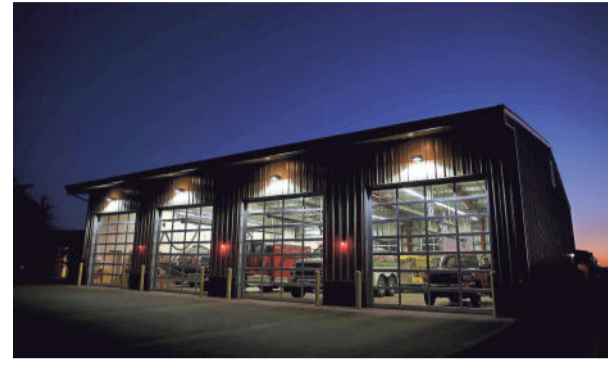
The Fire station located right next to the Chemeketa Community College Regional Training Center in Brooks on Wednesday, Dec. 5, 2018. Marion County Commissioners are looking at creating a special district for water in the unincorporated community of Brooks. MICHAELA ROMÁN / STATESMAN JOURNAL
