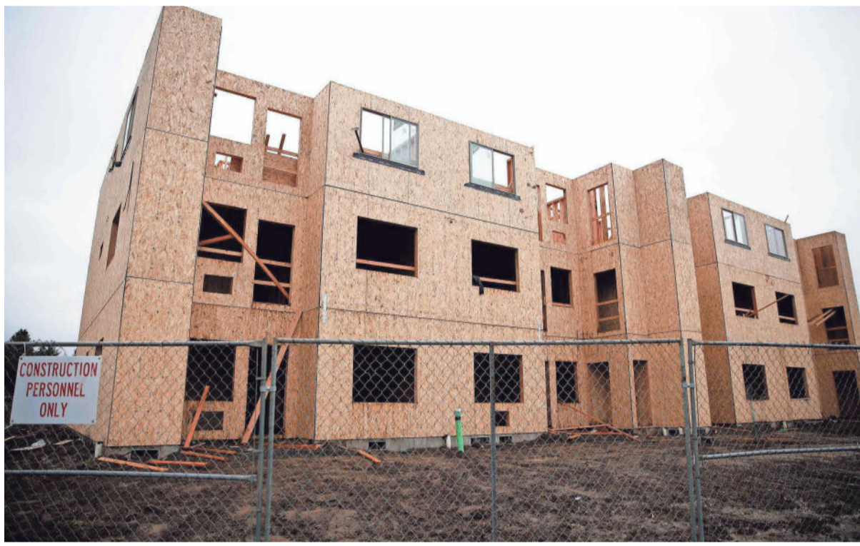
A 30-unit apartment complex is under construction in Jefferson on Jan. 22, 2020.
