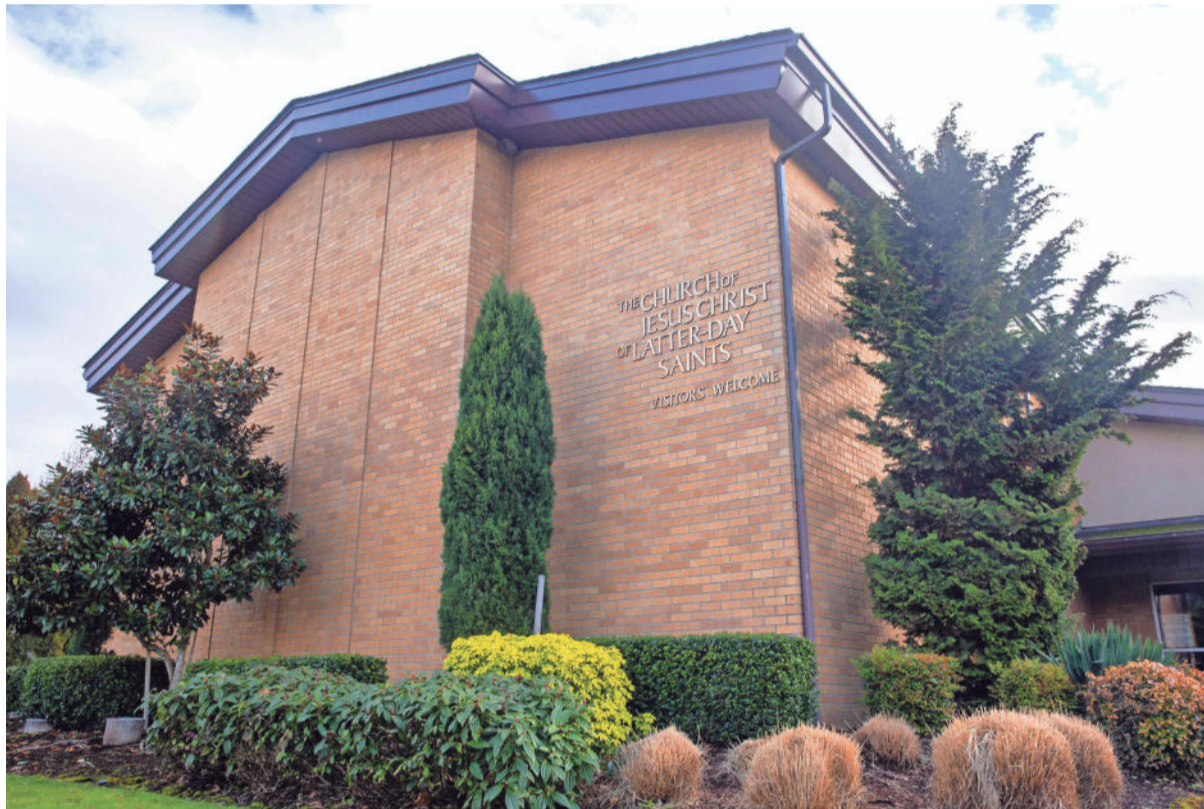
The exterior of the Church of Jesus Christ of Latter-Day Saints at 1400 Western Avenue in Stayton.
