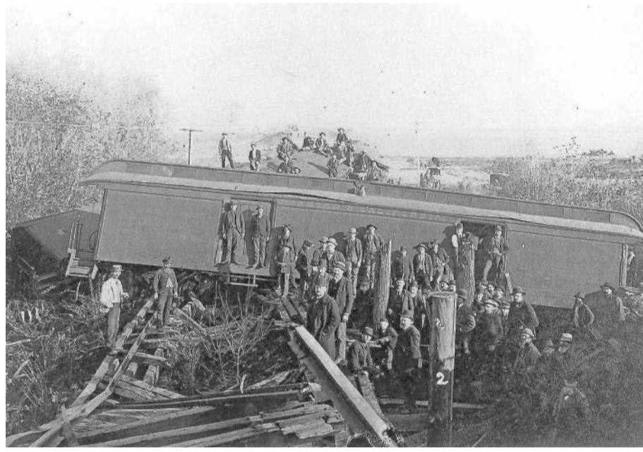
A Southern Pacific passenger train plunged through a dilapidated trestle at Lake Labish on Nov. 12, 1890. COURTESY OF THE ED AUSTIN COLLECTION
