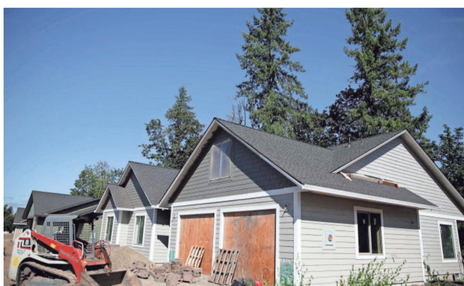
A small housing development under construction in Mill City on Aug. 15, 2019.
