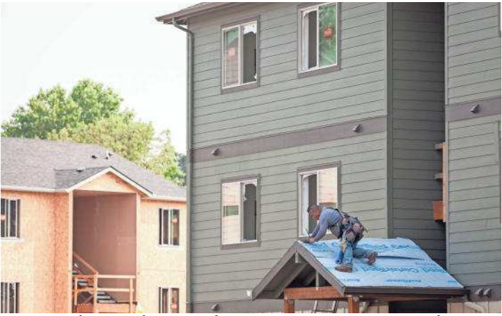
Construction continues at the Cornerstone Apartments in Salem in August. KELLY JORDAN/STATESMAN JOURNAL
