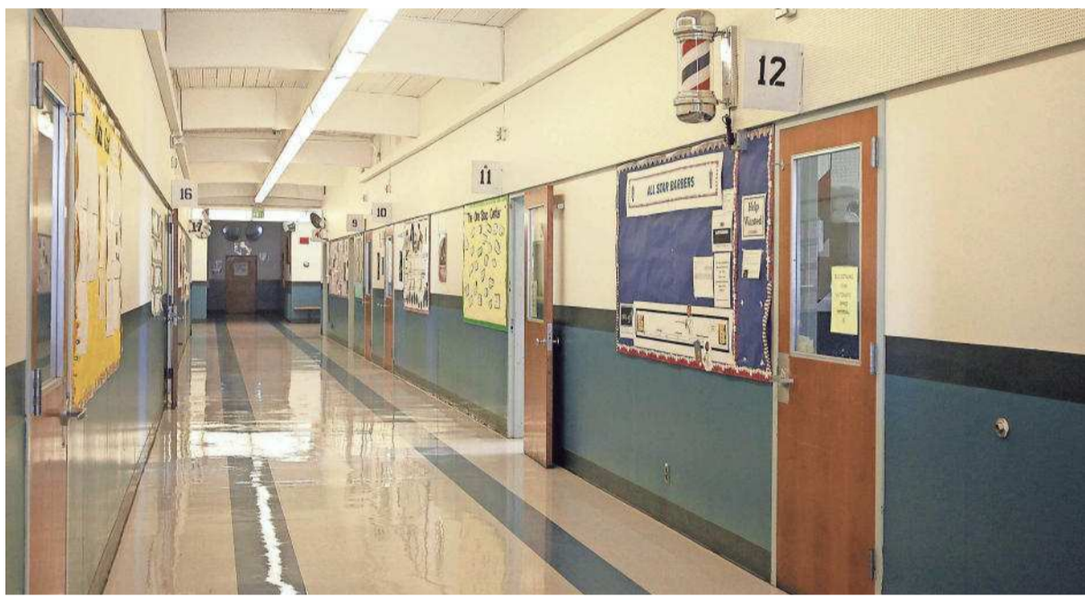
The hallways of Lord High School at MacLaren Youth Correctional Facility in Woodburn are shown in April 2014. The school was among eight buildings named in a lawsuit accusing the Oregon Youth Authority of knowingly exposing workers and students to asbestos. STATESMAN JOURNAL FILE
