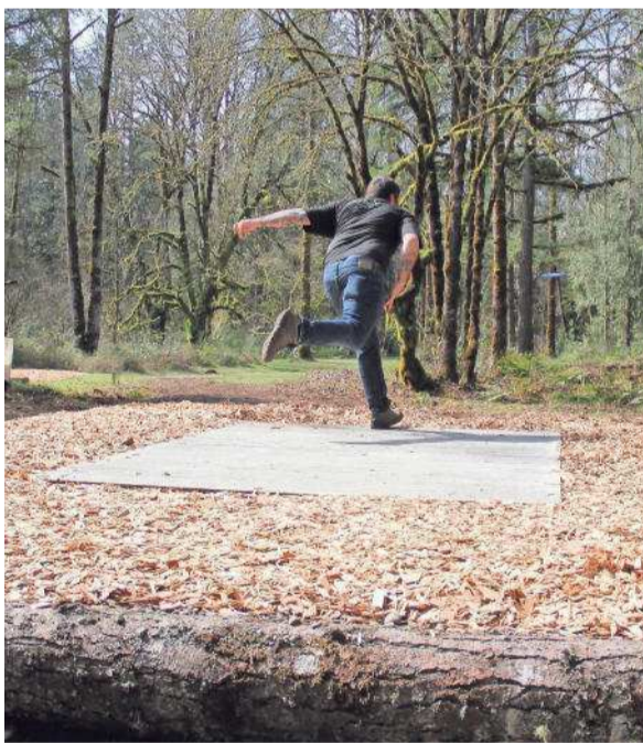
Matthew Coll throws a disc off the renovated tee box on hole No. 2 at the course.
