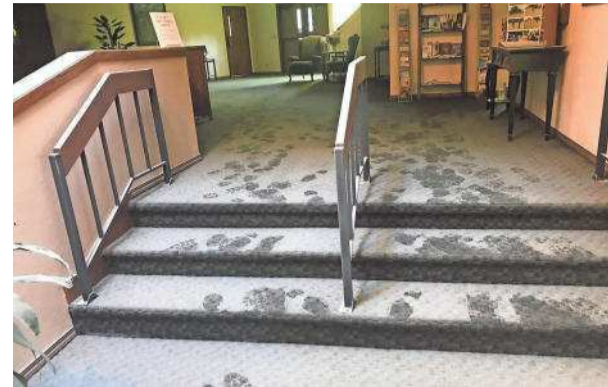
Fire extinguisher trails were part of the vandalism at the Silverton Community Seventh-day Adventist Church. The church was rendered temporarily unusable by the vandalism this month. PHOTO COURTESY OF OREGON CONFERENCE OF SEVENTH-DAY ADVENTISTS
