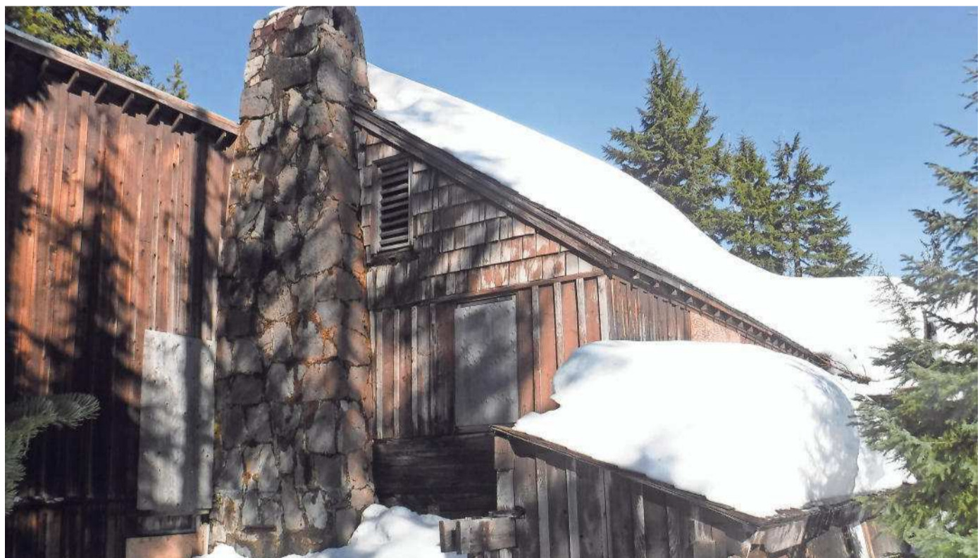
Santiam Lodge is covered in snow at Santiam Pass. This boarded-up, shake-sided relic was built by the Civilian Conservation Corps in 1939 and plans are in the works to restore the building.
