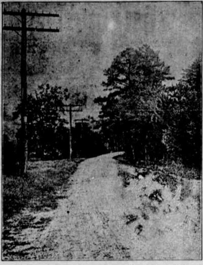
The illustration given herewith shows a "Tony Tank Road" in Wi comic county, Mich. It was built by the penetration method, with crush ed stone and "U. G. I. Binder."
