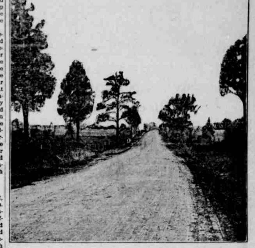
The illustration shows a modern oyster shell-macadam road between East Newmarket and Mt. Holly in the State of Maryland.
