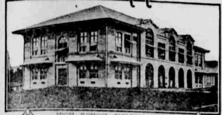
HIGH SCHOOL BUILDING, CEBU
