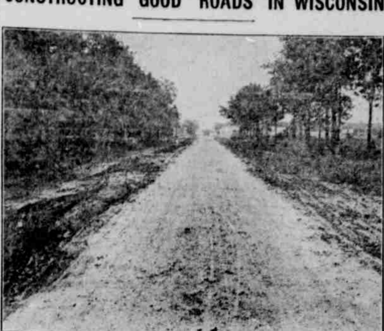
The illustration given above shows a nine-foot stone road, built on a sand foundation, near Portage, Wis.
