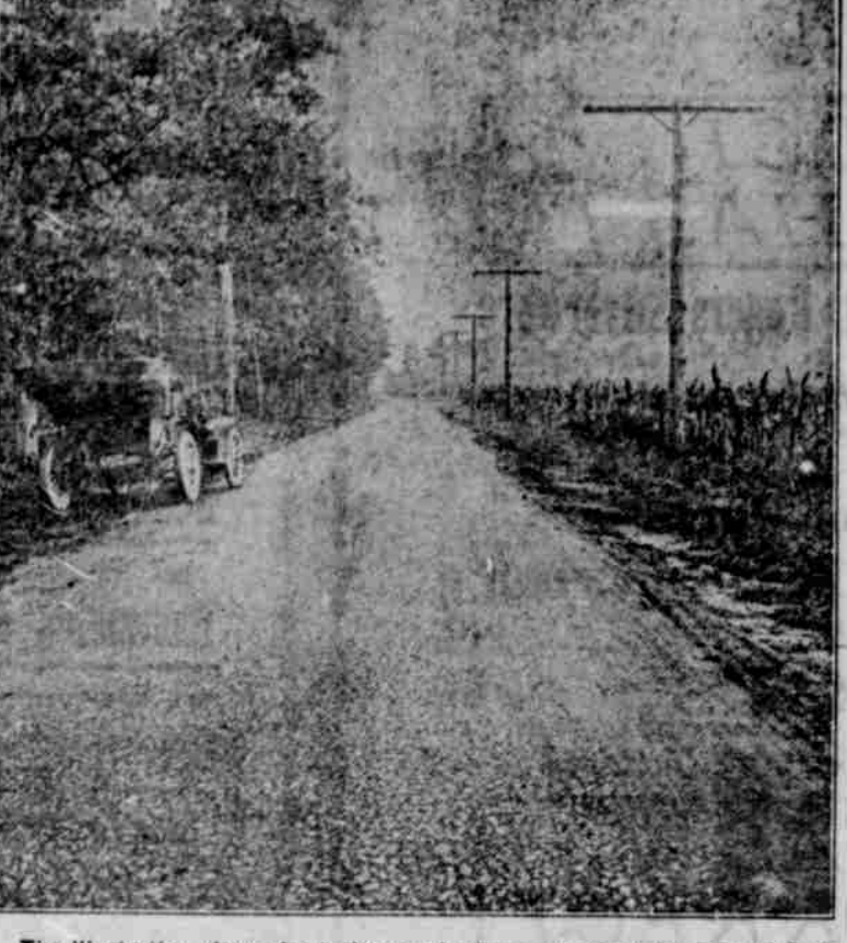
The illustration given above shows a broken-stone Macadam road, treated with "Texas 60 per cent" oil, near Salisbury, Md.
