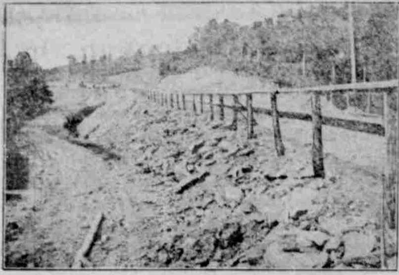
Piece of Heavy Grading Approaching Hill. New Grade, 8 Per Cent.; Old Grade, 16 Per Cent. Near Sparta, Wis.
