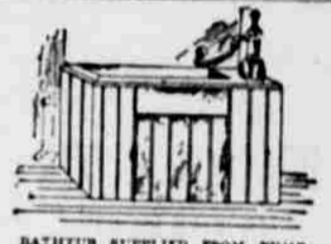
BATHROOM SUPPLIED FROM PUMP.
