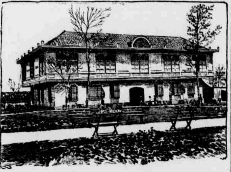
THE PHILIPPINE BUILDING, ST. LOUIS.
