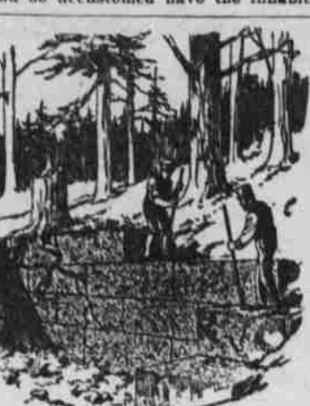
HISTORIC WALL UNCOVERED.
