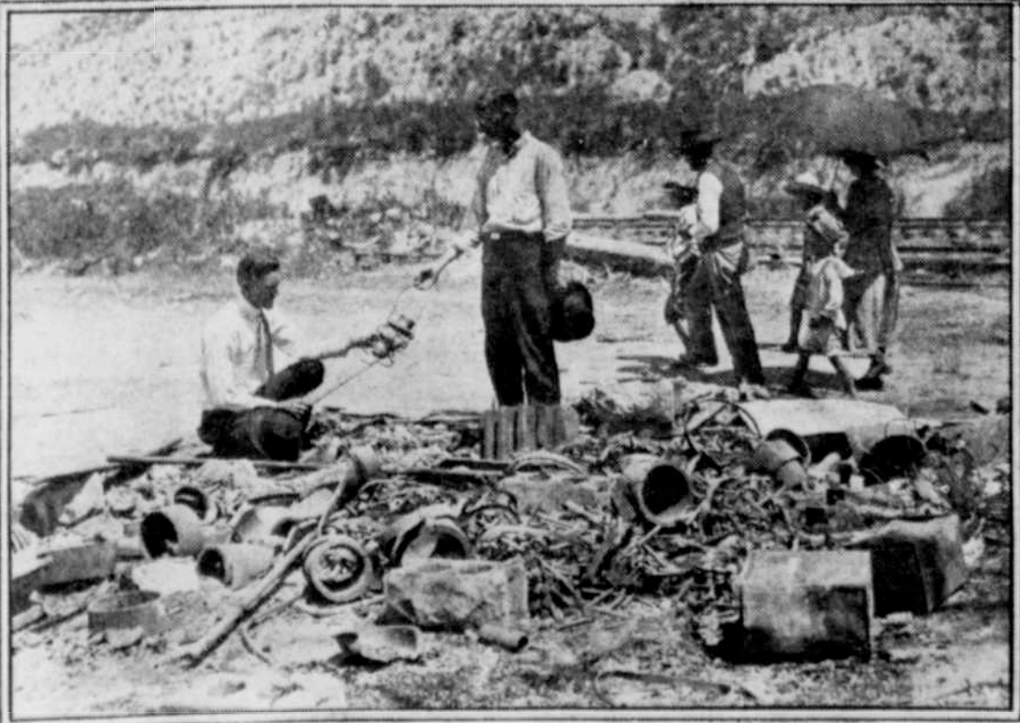
Photo shows all that remained of the supply house after the labor where a number of strike-breakers were killed recently. This building was dynamited and the job not suiting the miners they applied the torch.
