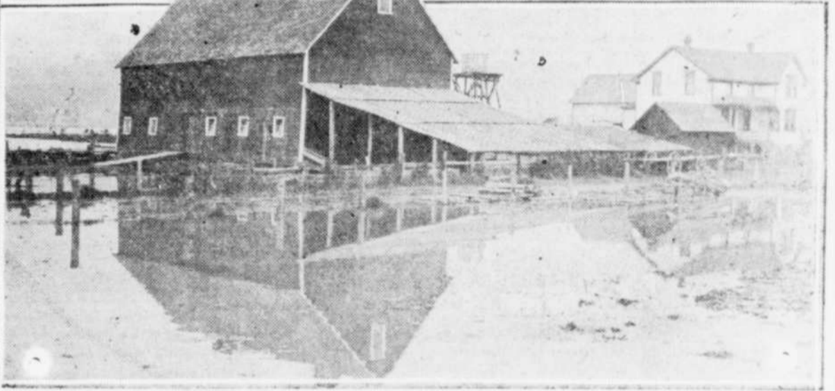
The pictures give some idea as to how the Columbia river demolished a portion of the Woodland dike. The upper picture was taken the morning after the dike broke at Burr's creek. The middle picture shows how the angry waters widened the breach and let the water into the thousands of acres of lowlands. The lower picture shows a farmhouse and barn which felt the effects of the flood. The lowlands were covered with water and the depth ranged from five to fifteen feet. No loss of life occurred, but several hundred head of cattle were drowned, and many of the farmers lost their crops.
