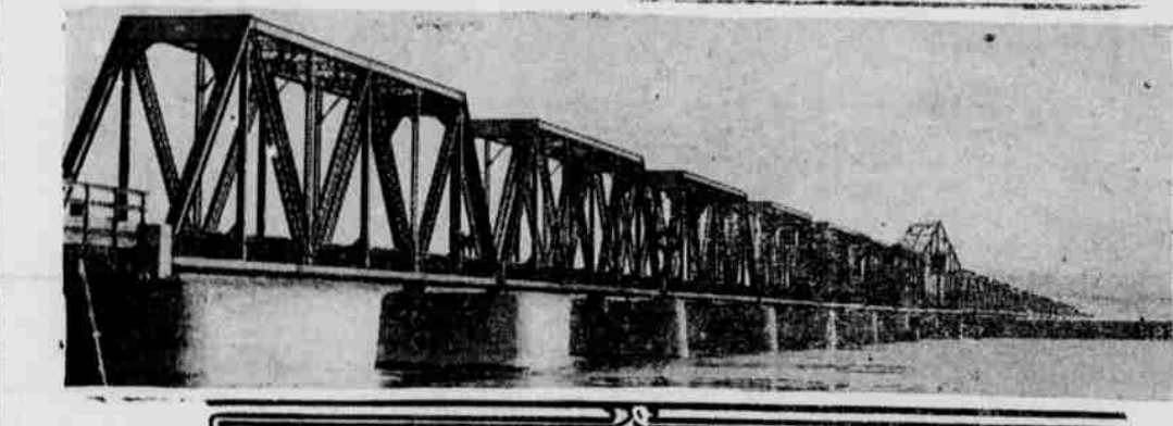
SOUTHERN PACIFIC BRIDGE ACROSS COOS BAY
