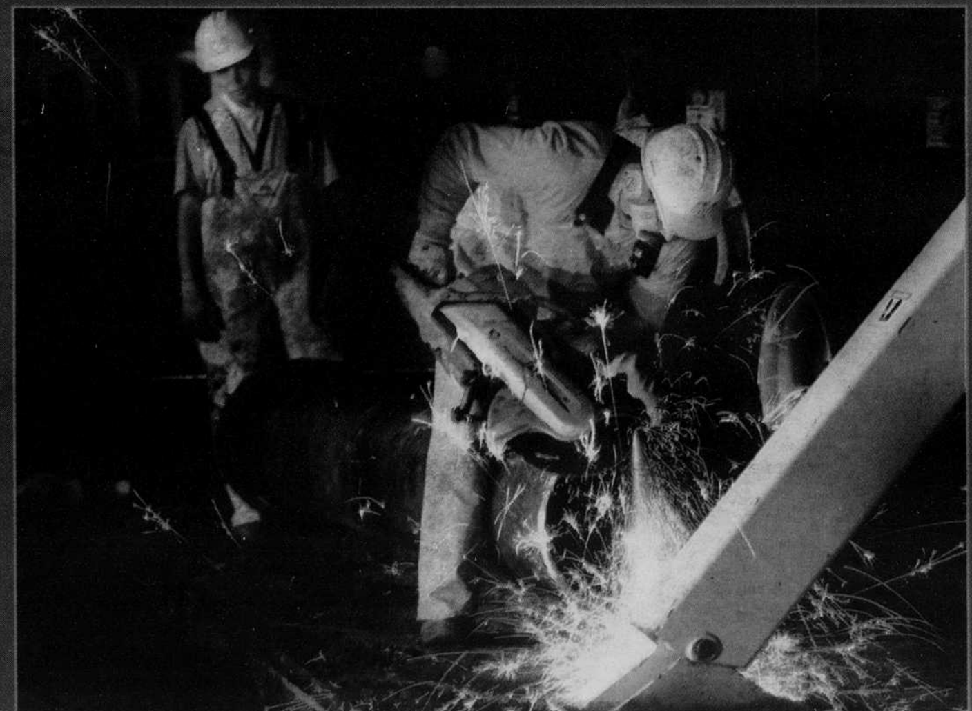
BELOW: Lisa Marie watches Craig Matsler (front) grind down the end to a replacement pipe March 28 in an effort to help repair the water main rupture damage at East 15th Avenue and Agate Street. Residents of Walton and Hamilton Complexes lived without water for about 24 hours because of the burst, which flooded the area. TIM KUPRICK | PHOTOGRAPHER
