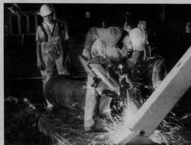
Worker Lisa Marie watches Craig Matsler (front) grind down the end of a replacement pipe for the burst water main.
