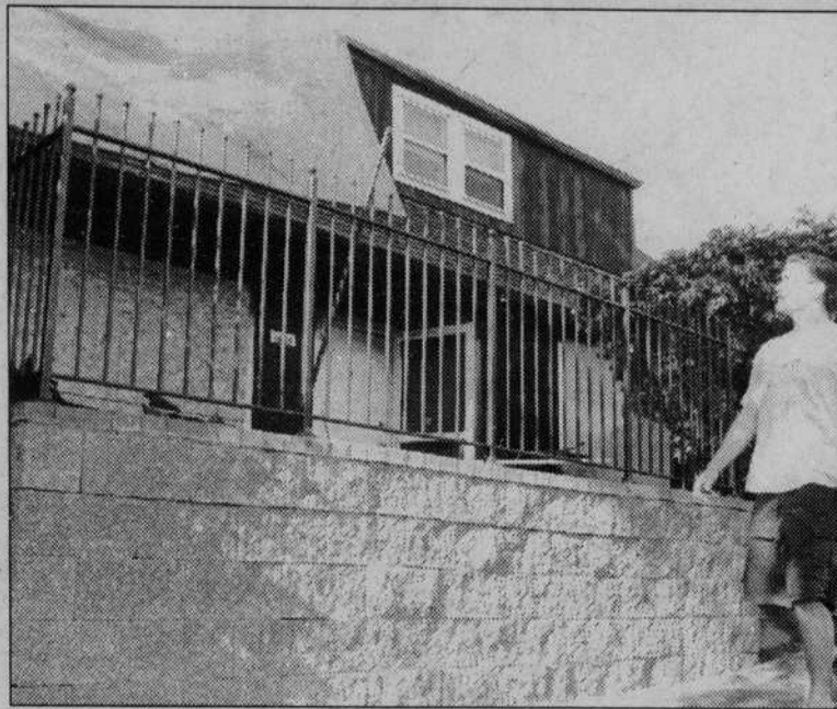
Danny Donaho walks past the fire damaged house at 1037 E. 19th Ave. The suspected arsonist struck in the pre-dawn hours Wednesday.
