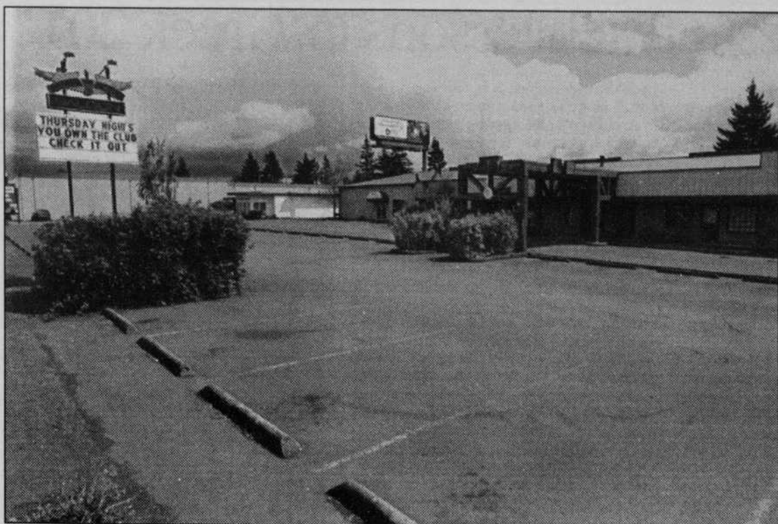
The Mill Camp Saloon on Q Street in Springfield will close permanently Saturday due to deterioration of the building. Scott Barnett/Emerald
