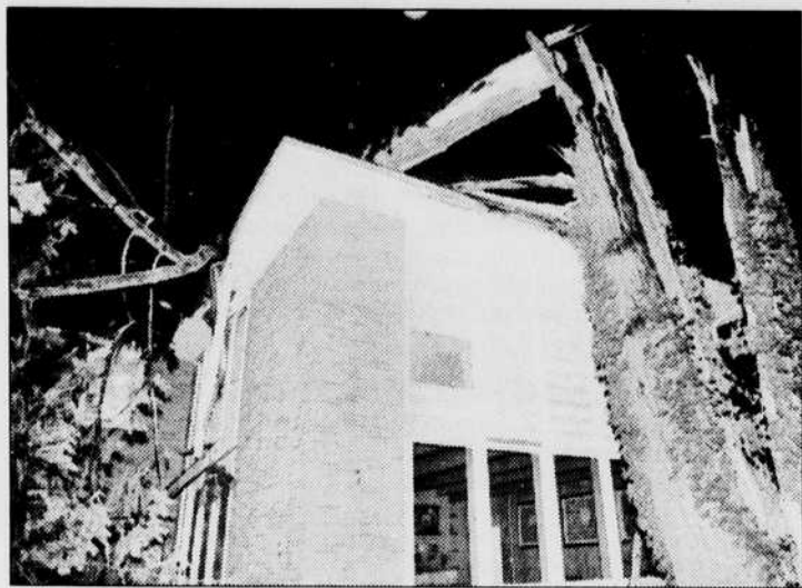
A tree fell onto the back porch roof of the Kappa Sigma fraternity house Tuesday night.
