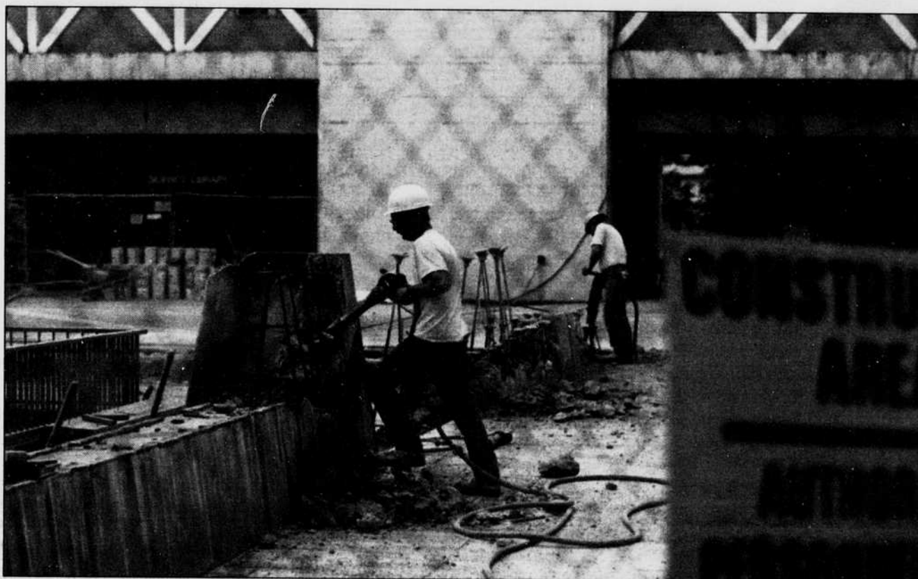
Workers started tearing up the plaza near Onyx Bridge last week to better waterproof the science library as well as adding handicap ramps and possibly covered bike racks. LAURA GOSS/ Emerald
