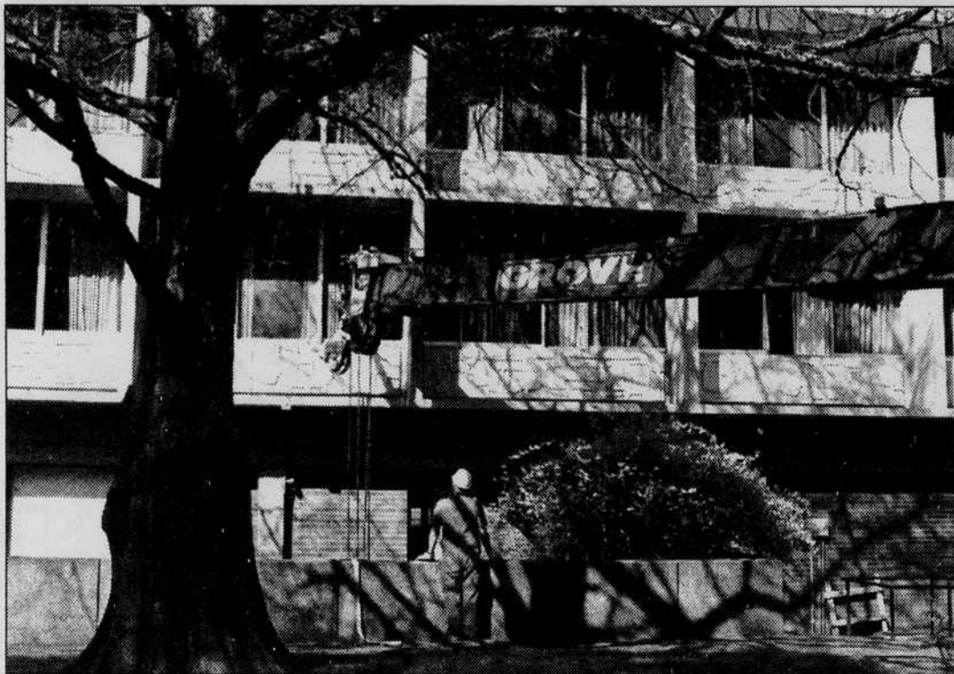
Gary Smith supervises the lowering of a new motor and compressor for Riley Hall's air conditioner. VERNON MICHAEL/Emerald
