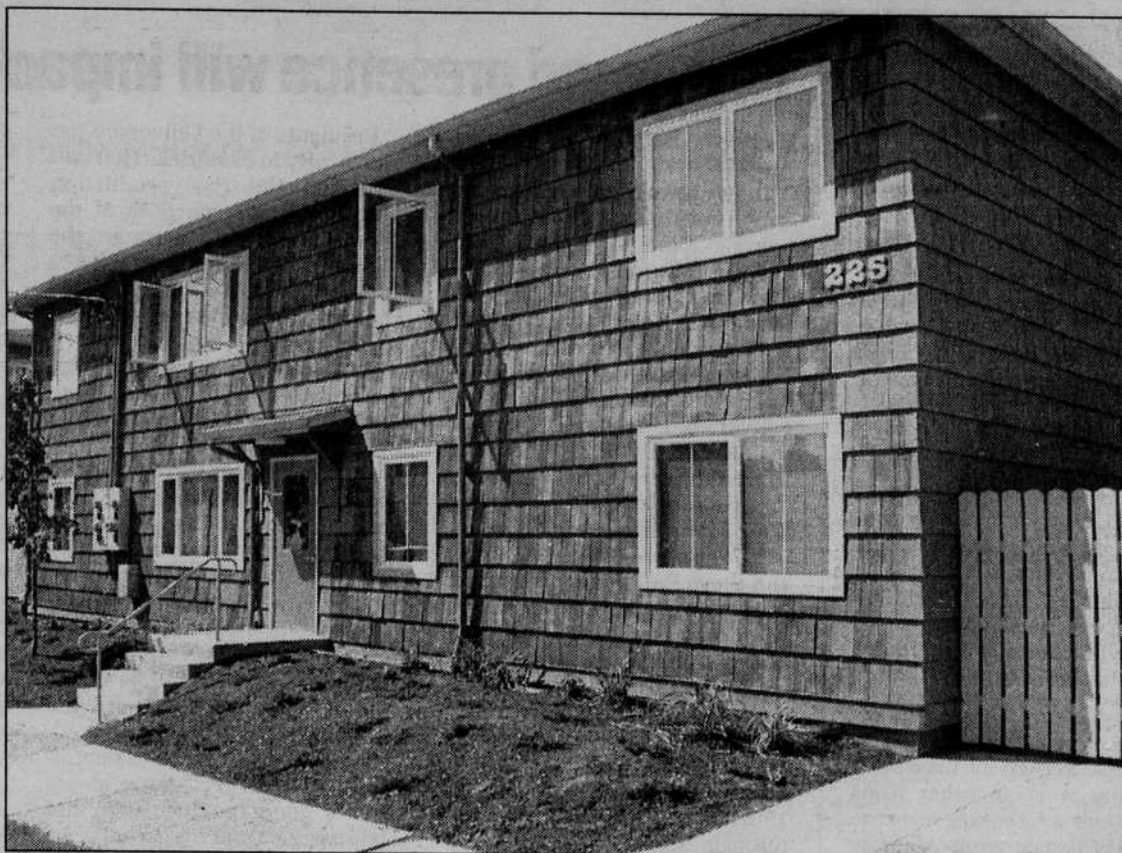
The newly renovated Bagley Downs apartments are some of the 30 Amazon buildings that were spared.
