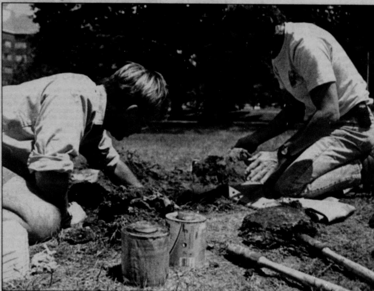
Repairing a broken irrigation pipe, Groundskeepers Miguel Rementeria (left) and Rick Green patch a punctured pipe beneath the EMU East Lawn. The pipe was damaged after an aerator machine dug too far into the ground. Aerating the lawn is one of the methods that the grounds crew is using to repair the area that was damaged from heavy rain and traffic during the Willamette Valley Folk Festival.
