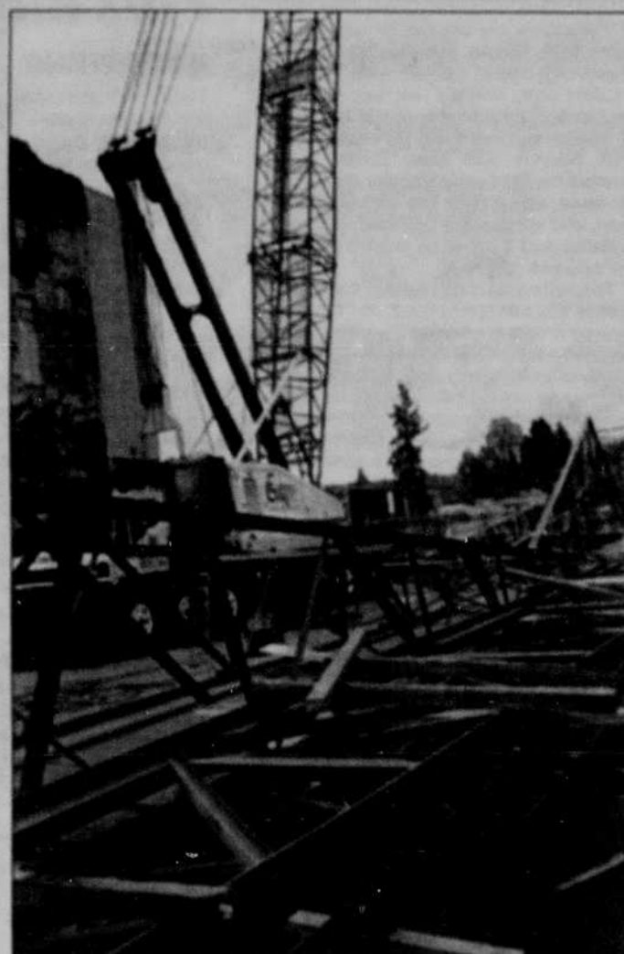
Support beams and the crane used to place them sit quietly while the University waits for building permits to arrive.
