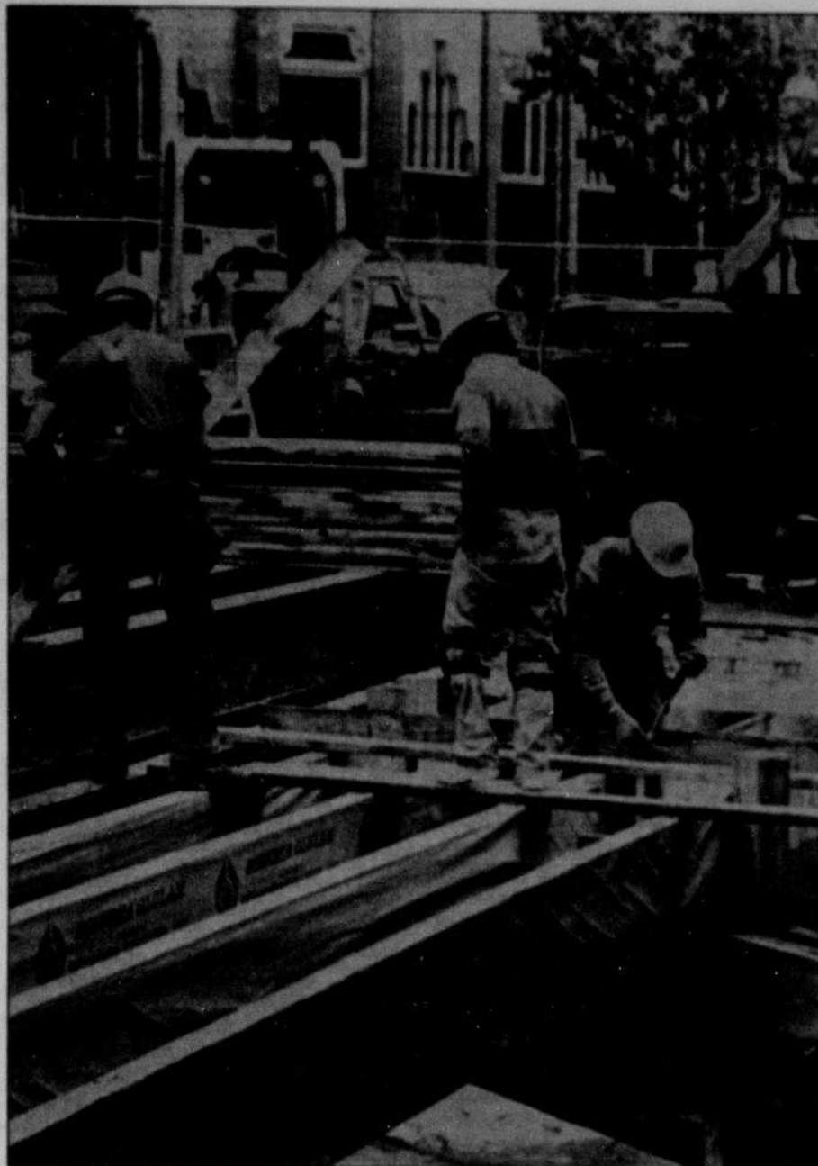
The demolition of the fountain isn't the only construction work being done downtown. Workers place beams to support the street over a tunnel that will connect the Downtown Athletic Club and its day care center across the street (above). At the other end of the mall, construction crews have begun to fill in the sunken courtyard in front of the Aster building on Willamette Street.
