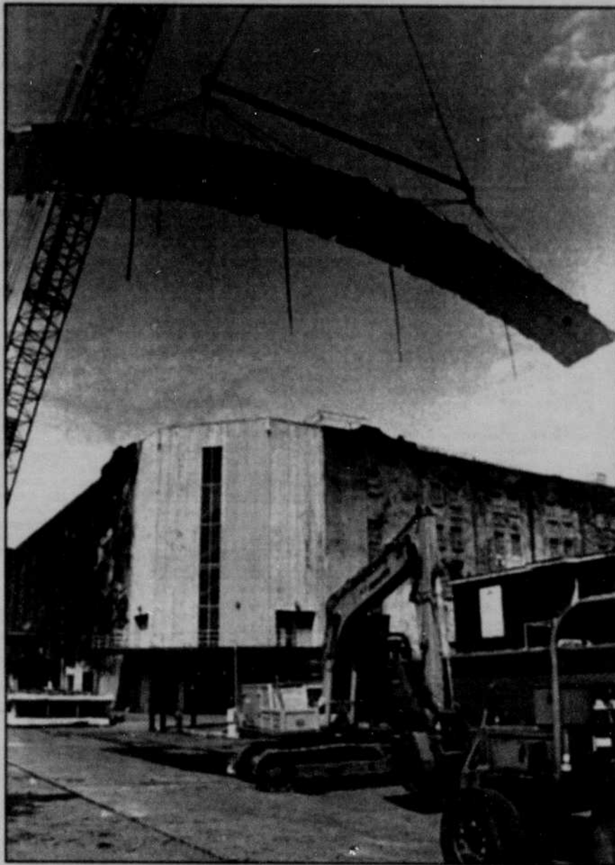
At thousands of dollars a day, a 250-foot mobile crane removes a piece of McArthur Court's wooden-barrel roof Wednesday afternoon. The crane also will be used to maneuver 17 steel roof trusses for the new gable roof.
