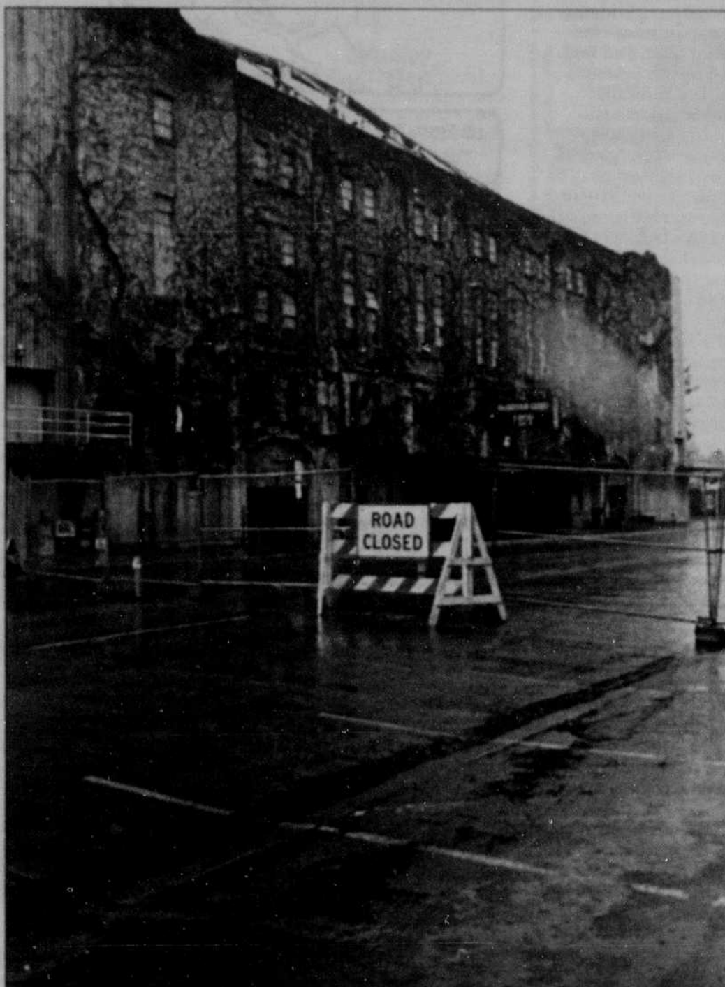
Drivers turning onto University Street will be greeted by a "road closed" sign during spring term, as workers replace the roof on McArthur Court. The closure has resulted in the loss of about 120 parking spaces, although 48 replacement spaces have been opened south of Agate Hall.
