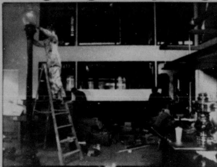
Workers rush to finish construction of the Wild Duck, a new bar co-owned by a former UO quarterback, which is scheduled to open today.
